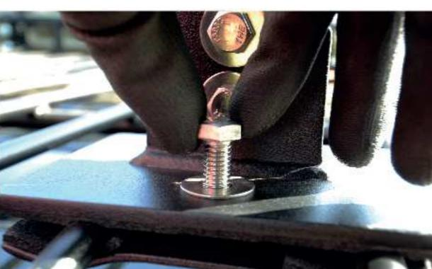
Place the Holding plate (B) below the Base plate (A). Insert washers (D) and bolts (C) in the base plate holes, then, inserting washers (D) and nylon lock nuts (E) in the bolts (C).
