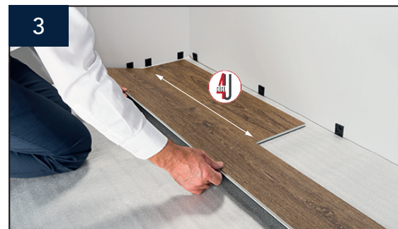
Figure 3: Use a full length for Plank 2 which will be installed in the second row. Align plank 2 at an angle, onto the long side of plank 1 making sure there are no gaps. Drop plank 2 to lock in place.
