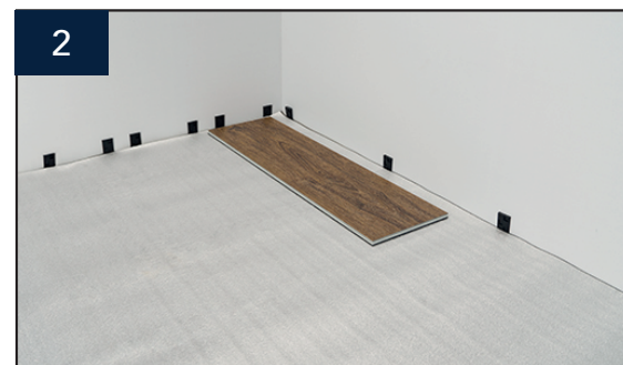
Figure 2: Begin by cutting plank 1 in half. Position the cut end of plank 1 against the wall in the left corner of the room.
