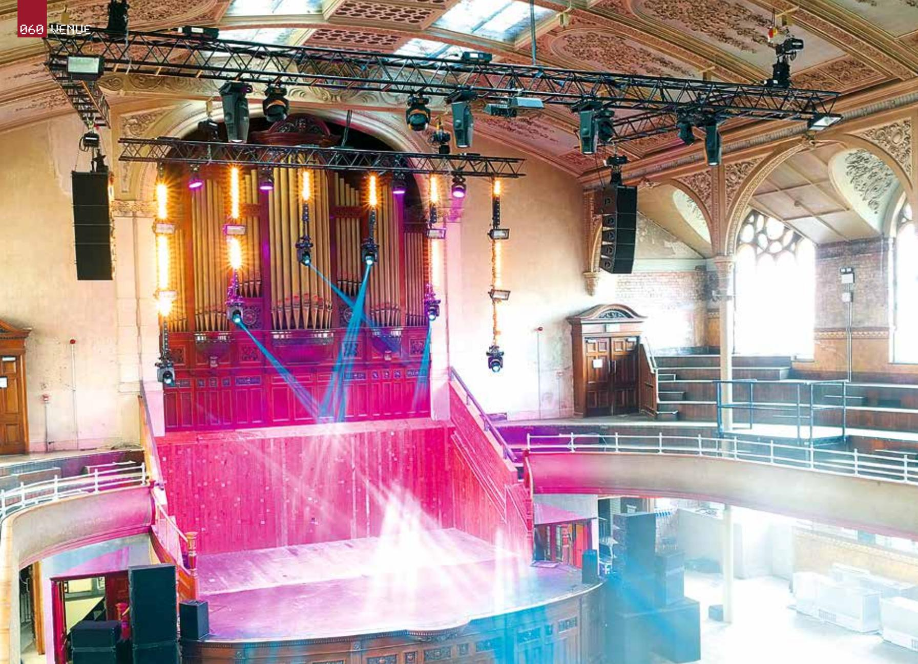
needing additional safeties, which is essential as roof access at Albert Hall is difficult given the height and construction of the venue. The motors are top hung and LTM has down-rated the clutches to further protect against overloading of the roof structure.
