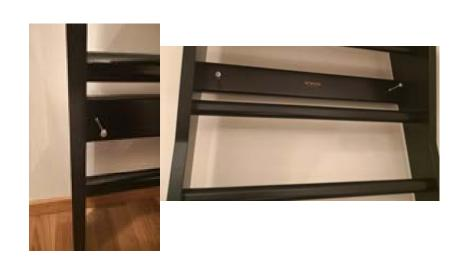
Lift the Wall Bars to its correct place. Ensure that you have marked the correct location for the fastening wooden mounting rails. Also, make sure to use proper and safe connection to studs or other type of wall structure.
