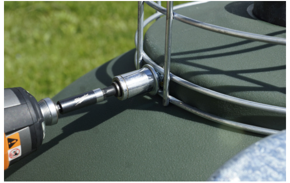
Step 6: Bolt cage to unit.
