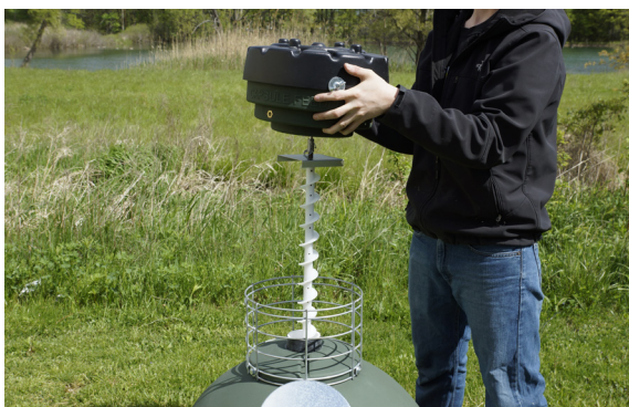
Step 9: Place powerhead on top of cage.
