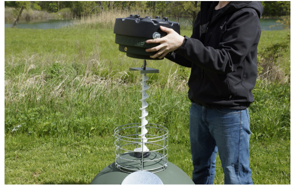
Step 10: Place powerhead on top of cage.
