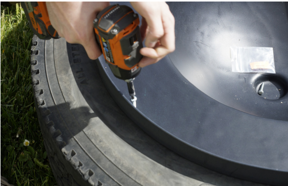
Step 3: Attach base to tire. (4) Tire screws
