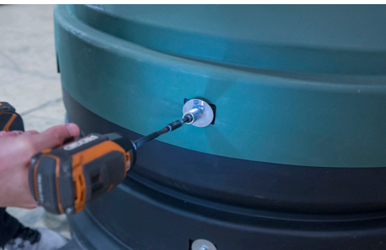
Step 7: Attach dome to extension ring.
