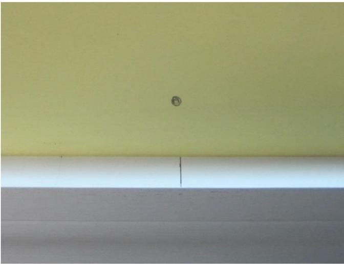
Mark the wall through the hole in the center of the backing plate.
