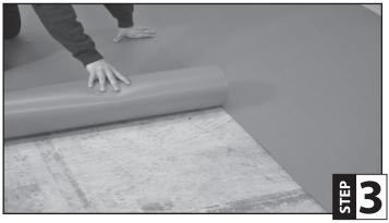
**Step 3:** Roll out the next roll of FloorMuffler® in the same manner making sure that the foam seams are butted together.
