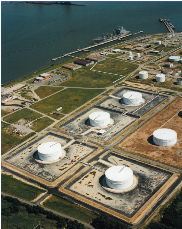
Figure 6.3 A compartmentalised bund (courtesy Seaman Corporation)
