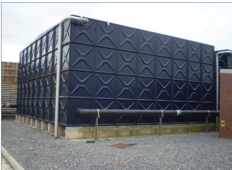
Figure 9.2 A pressed steel sectional rectangular tank (courtesy of Braithwaite Engineers Limited)
