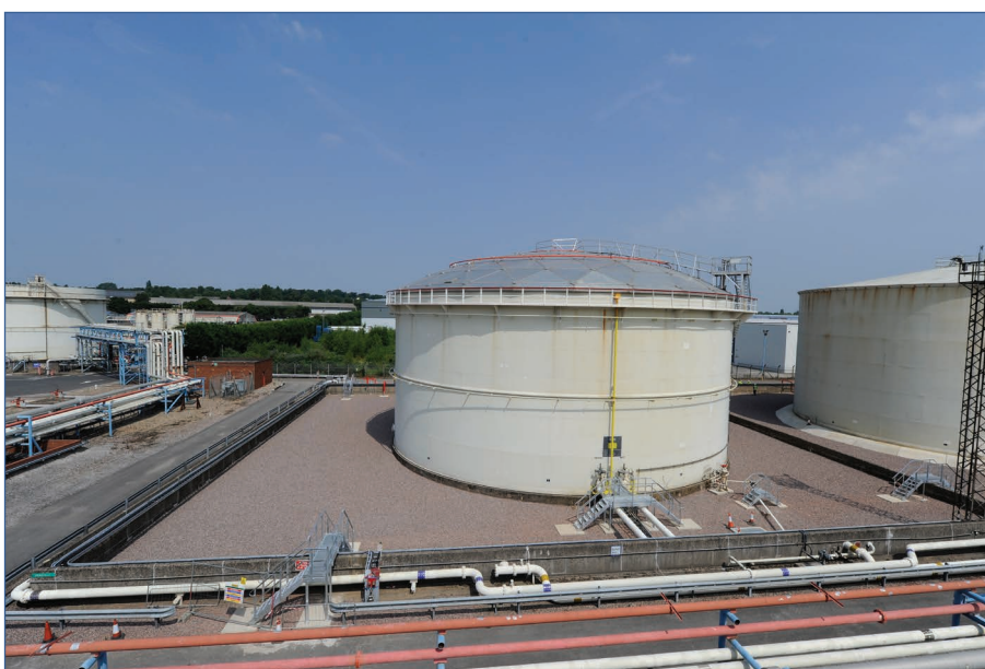
Figure 6.1 A bunded tank farm (courtesy Steve Flynn, Rawell Environmental Ltd)
