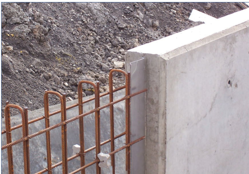
Figure 5.10 A metal waterstop in a wall joint (courtesy Environment Agency)
