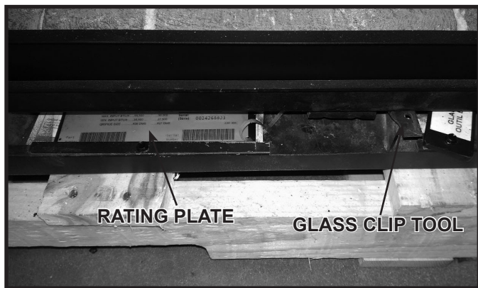
Figure 3.3 Rating Plate/Glass Clip Tool Location
