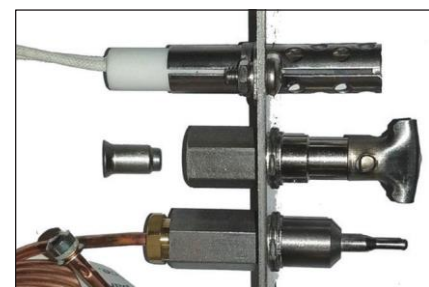
Figure 9.3 – Cleaning pilot orifice
