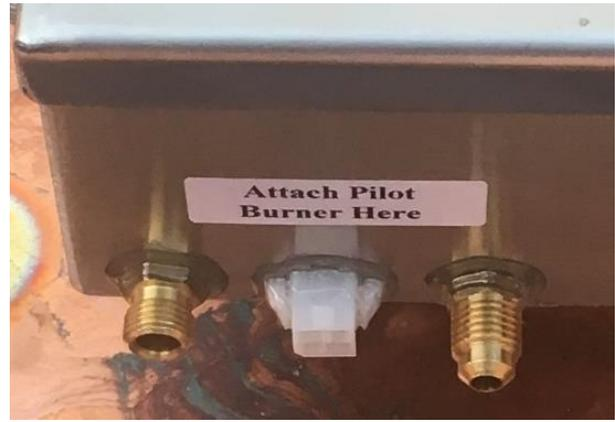
The photo at right shows the AWEIS after the Pilot Burner Assembly has been connected. Notice the Brass Compression Fitting on the left and the Brass Flare Nut on the right.
