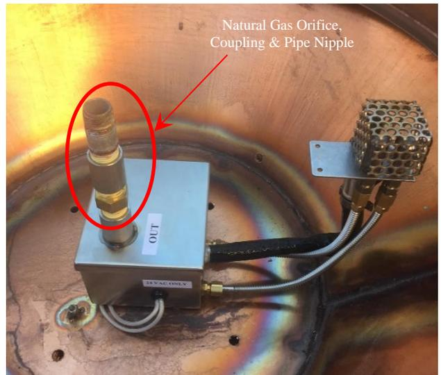
6. Install the Burner Pan. You will need to line up the Opening for the Pilot Burner with the Pilot Burner. You will notice that the hole in the center of the pan (for the pipe nipple coming from the Ignition Control Box) and the opening for the Pilot Burner are much larger than needed. This is done to make it easier to Install the Burner Pan. The large gaps around the pipe nipple and Pilot Burner will be covered with additional parts sent with the Burner Pan in Step 8 and 9 below.
