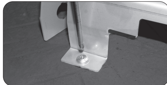
Fig. 15-2 Fastening hammer screws
