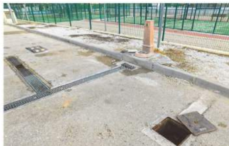
Lift up covers are common for toilet waste disposal
