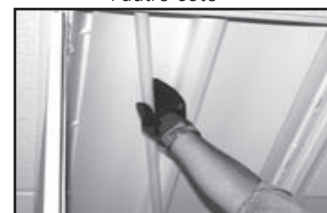
Figure 8. Installation des lampes
