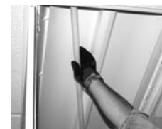
Step 5. Inserting supply wires into quick disconnect
