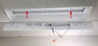
Install tether cable to lighting fixture housing using self-tapping screws at two places.
