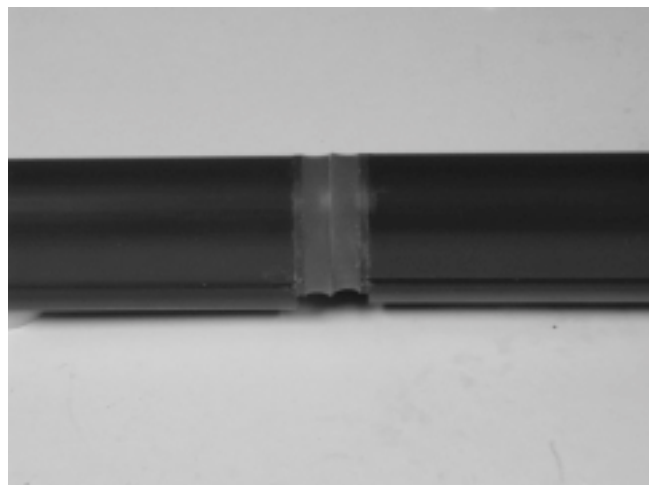
Finished connections with wires and connector hidden in mounting track Figure 11
