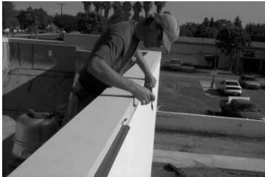
Marking the mounting button location
