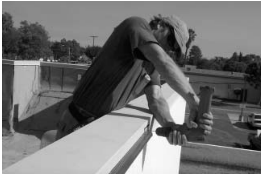
Drilling mounting button holes for an BriteStripe section Figure 4
