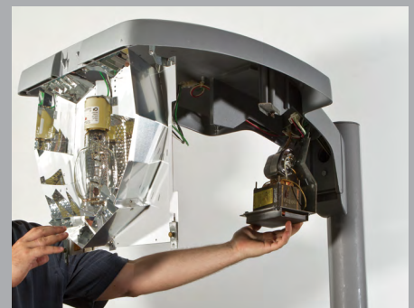
Remove the existing HID reflector system and ballast tray.
