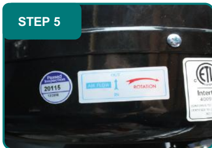
Note the direction of airflow in the fan
