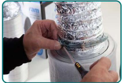
Slide the ducting over the flanges and secure
