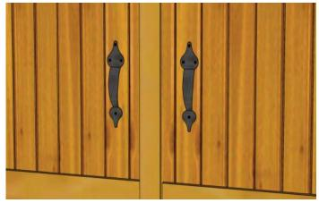
**63.** Attach **Door Handles** to Doors with **4 - 3/4" Black Headed Screws** per Handle. Choose desired Handle height.
