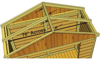
**32.** At the peak, align Ridge Boards so they are flush together and secure them with **4 - 1 1/4**" **Brown Screws**. **Important:** If there is a gap between Ridge Boards, have a helper push the Side Walls closer together from outside. Walls should be 70" apart at top from inside of Wall plate to opposite Wall plate.
