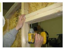
Also insert 2 1/2" screw from bottom of header up into 2x4 as shown.
