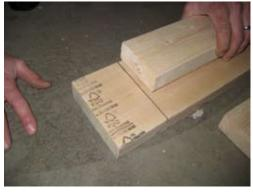
Lay out 2x6 and screw 2x4 on top. Stay even with pencil mark.
