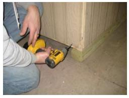
Next secure the bottom edge all the way around with 1 1/4" screws 8" on center.
