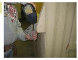
Make sure all four corners are flush on outside of top plate as shown.
