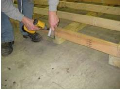
Next make sure 4x4's are positioned in place and secure with 2 1/2" screws as shown.
