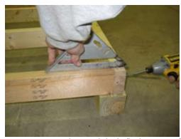
Use square to make sure joist is flush on top of rim as shown and secure with 2 1/2" screws.
