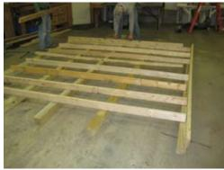
Next layout 2x4's for floor joist.
