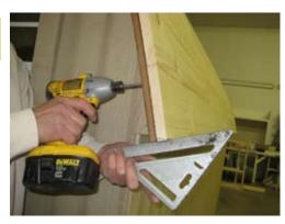
Use square to make sure rafter trim is flush on bottom as shown. Secure with 1 1/4" screws.
