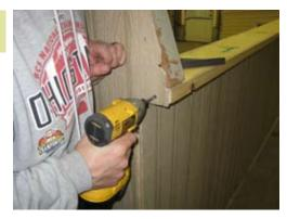
Insert 1 1/4" screw through siding into 2x6 Top Plate.
