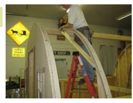
Install top first and secure with 2 1/2" screws.
