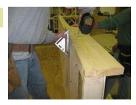
Continue with top plates and make sure it is flush on inside as shown.
