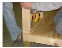
Apply Pressure on outside and secure with 2 1/2" screws.
