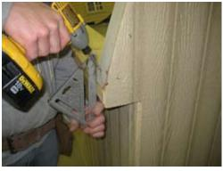
Make sure rafter is flush with 2x6 top plate and secure with 2 1/2" screws.
