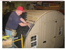
Make sure shingles are cut off at 1/2" over the edge of the roof.
