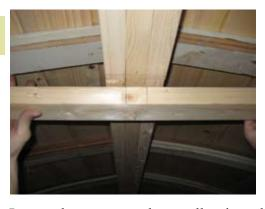
Locate the center mark on collar tie and make sure it center with 2x6 as shown. Secure with 2 1/2" screws at center and each end.
