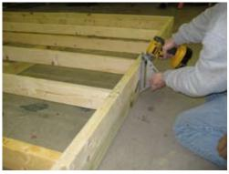
Continue all the way out around as shown so 2x4 is flush with 4x4 and secure with 2 1/2" screws.
