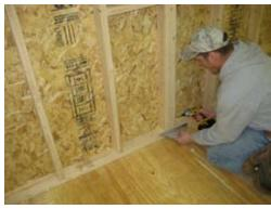
Insert 3 to 4 2 1/2" screws, where 2x4's meet to tie wall together.
