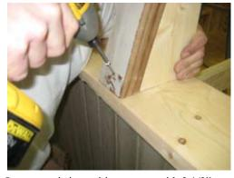
Once truss is in position secure with 2 1/2" screws.
