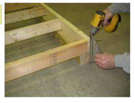
Next make sure 4x4 is flush with rim as shown and secure with 2 1/2" screws.
