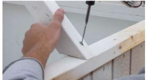
Set rafter in place and secure using a 2½" screw. Repeat on opposite side.
