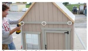
Secure trim to front of structure using three (3) 11/4 black headed screws as shown above.
