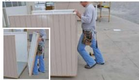
Locate rear panel, set in place, and apply pressure to ensure proper fit between side panels. Secure along the bottom (inside) 2X per step #2.
