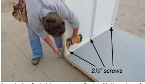
Locate the first side panel, set flush with the edge of floor, and secure by driving a 2½" screw through lower plate and into floor. Additionally, drive screws at the opposite corner and at the center 2X.
