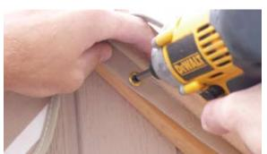
Secure roof covering by driving 1¼ black headed screws through each eyelet and into roof framing.
