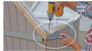
With front and rear gables now in place, locate and set rafter plates. Using an angle to ensure that the edge of plate is flush with the end of gable, secure using a 2½" screw.
