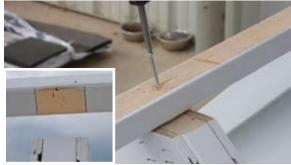
Align center rafter with mark on underside of ridge beam (see inset) and secure using a 2½" screw.
