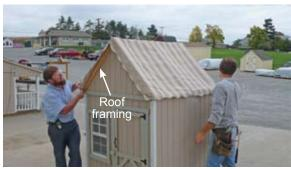
Align roof covering on all sides, ensuring that the front and back (as well as both sides) equally overhang the roof framing.
