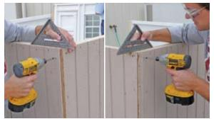
Verify that top corners are flush and drive 2½" screws at top (as above), in the middle, and at the bottom of corners.
