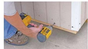
Secure siding along bottom of structure by driving 1¼ black headed screws every 8" (all sides).
