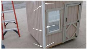
Locate and set corner trim on all corners as shown using three (3) 11/4 black headed screws per side.
