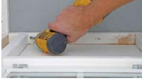
Locate front panel, noting that door and window are preset. Set panel in place and secure to floor using 2½" screws at each corner and beside each 2X.
