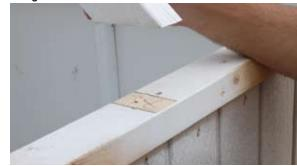
Locate center rafter and align as marked on the rafter plate.
