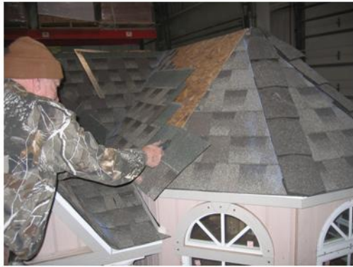
Cut shingles to fit each section.
