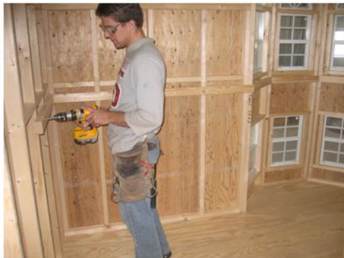
Continue to install the loft braces.
