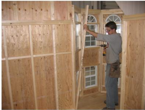
Place 2x3 on end of O-panel on inside.
