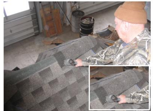
Fasten ridge cap as shown.
