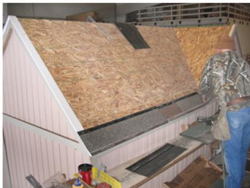
Layout your starter strips and fasten.
