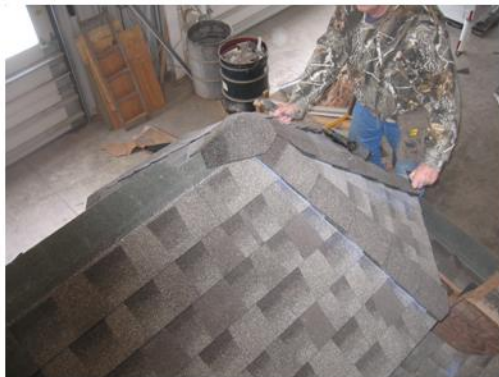
Install ridge caps along each peak...
