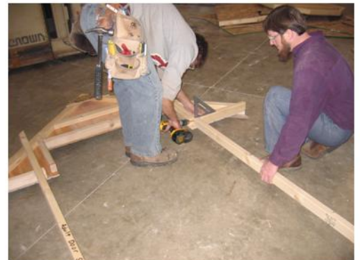
Install the 2x3 door studs on the R-panel. Fasten with 2 1/2" screws.
