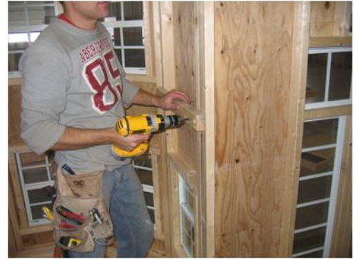
Install loft braces and fasten with 2 1/2" screws.
