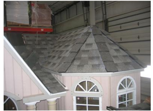
Ridge caps are being installed.
