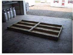
To begin construction of your Cape Cod playhouse simply lay out (2) 4x4 flooring sections side by side. Make sure it is on a level area.
