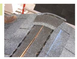
When you have done both sides, cut caps for the peak of the roof. To cut "caps" cut the tabs. For Example: If there are 3 tabs per shingle there will be 3 "caps", just continue to cut the line through the shingle.
