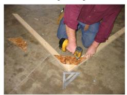
Fasten the truss gussets, keep the top even. Use zinc screws for this. Install one gusset on either side of the truss. For a total of 2 per truss.
