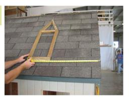
Check the layout diagram for correct measurements for your size building. Measure from the edge of the building to edge of the treated dormer frame. There is a cut angle right where the fingers and tape are in the picture. Make sure this angle is turned up and not down toward the roof.
