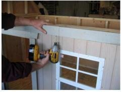
Fasten the 1x3 to the center section using zinc screws. This will straighten the 2x6 and make it strong.
