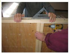
Install panel G. Fasten in corner and bottoms as shown before.
