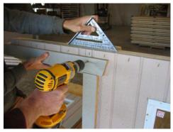
Now make sure it is even on top. Fasten the trim on the header block B into the siding.
