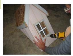
Install pre drilled dormer grid window trim.
