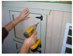
Next install the top door piece. Try to center the door between the header block and the bottom door. If both doors work well, install the rest of the screws and remove spacer bar.
