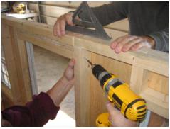
Install panel C. Fasten this onto the header block as shown.
