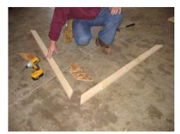
Lay trusses as shown. On the 4x6 and 6x8 sizes, the trusses are the same angle. On the larger sizes (8x8, 8x10, and 8x12) the angles are different on one end. Make sure the correct angles are matching. You can check this with the gusset angles.
