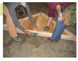
Assemble panels H and I. Make sure they are even on the bottom . Fasten.
