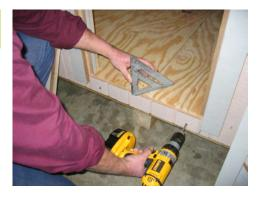
Install a siding piece below the child door and the adult door. Be sure to keep level with the floor.
