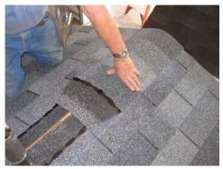
Install the caps as shown. When you reach the end you can use only the exposed part of the shingle to give it a nice finish. For Example: The cap would then be cut in half for this.
