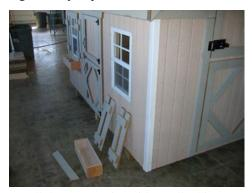
Install the corner trim with small white nails. Be careful to not "wrinkle the corners" when installing.
