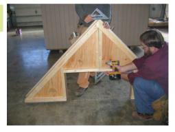
Fasten panels L & M together. Note to keep the bottom edge even. This will be the top of the door so it is very important.
