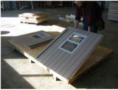
Install section A BE SURE to install the trim toward the center as shown! This is the trim for the small door. This is the start for a 6x8 other sizes are slightly different. The same basic structure is used. Refer to the wall layout documents for the alphabetical order.
