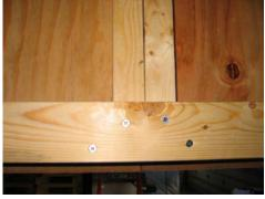
Install screws as shown over joints. This provides strength for joints.
