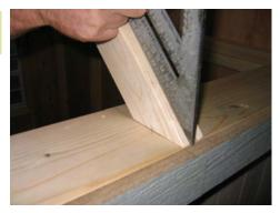
Truss should fit as shown. Make sure truss does not go past the edge of the 2x6 onto the trim.
