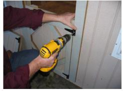
Place the door on the spacer bar. Fasten using only one screw per hinge. This way if adjustments are needed you will not have to undo all the screws. Use zinc screw for these.
