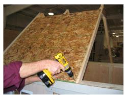
Install first sheet of OSB (orient strand board) sheeting. Fasten only on the bottom first. Refer to layout diagram for your specific building. Use zinc screws to fasten.
