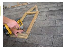
Screw the bas into the roof. You can use 2 1/2" screws. Be sure to check on the inside and break off the screw that is exposed.
