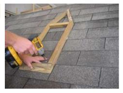
Screw the bas into the roof. You can use 2 1/2" screws. Be sure to check on the inside and break off the screw that is exposed.
