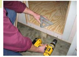
Install a siding piece below the child door and the adult door. Be sure to keep level with the floor.
