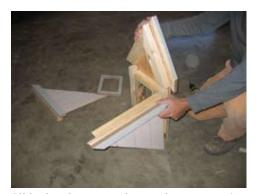
Slide the pieces together as shown. Use 2 1/2" screws to fasten together.
