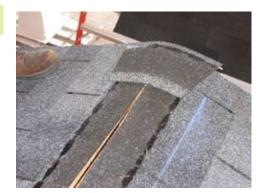
When you have done both sides, cut caps for the peak of the roof. To cut "caps" cut the tabs. For Example: If there are 3 tabs per shingle there will be 3 "caps", just continue to cut the line through the shingle.
