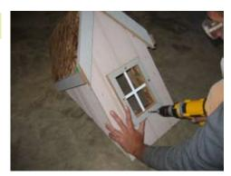
Install pre drilled dormer grid window trim.
