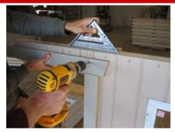
Now make sure it is even on top. Fasten the trim on the header block B into the siding.
