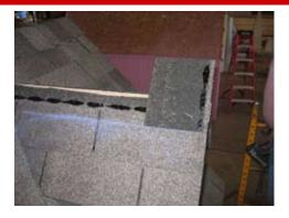
Start by installing a starter cap.
