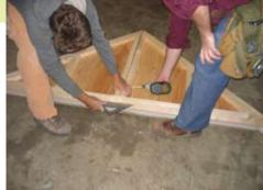
Assemble panels H and I. Make sure they are even on the bottom . Fasten.
