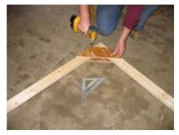
Flip the truss and install gusset on other side.
