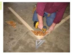
Fasten the truss gussets, keep the top even. Use black headed screws for this. Install one gusset on either side of the truss. For a total of 2 per truss.
