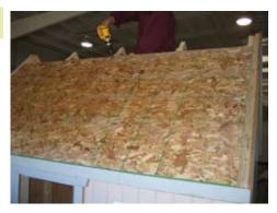
Note gap between OSB and 2x2 with trim. Be sure you have this before fastening on top.
