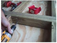
Screw the sections together. Put one screw towards the plywood, and the other toward the top. Put 4 screws on each side roughly 8"-10" apart
