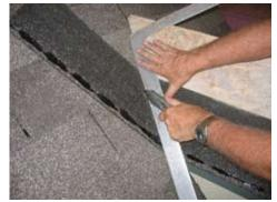
Cut the excess past the dormer. Be sure to use a hook blade so you do not cut into the other roof shingles.
