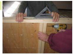
Install panel G. Fasten in corner and bottoms as shown before.
