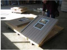
Install section A BE SURE to install the trim toward the center as shown! This is the trim for the small door. This is the start for a 6x8 other sizes are slightly different. The same basic structure is used. Refer to the wall layout documents for the alphabetical order.
