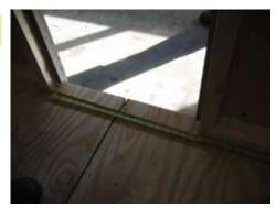
Be sure to measure from 2x3 to 2x3 that the opening is 20". Do not measure in between the door stop. If it is not you may need to adjust it one way or the other.
