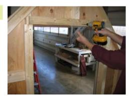
Install (3) 2x3x36" pieces over the top of the door and sides over joints. This will provide strength for the door. Keep even with the edge of the door.
