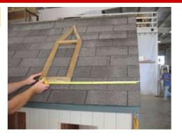
Check the layout diagram for correct measurements for your size building. Measure from the edge of the building to edge of the treated dormer frame. There is a cut angle right where the fingers and tape are in the picture. Make sure this angle is turned up and not down toward the roof.
