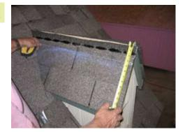
Once the last row is installed measure 4 1/4" from the top down and snap a chalk line. This ensures a straight line for the cap.
