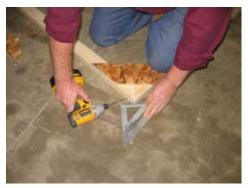
Keep the top of the truss even and install 2 1/2" screws as shown.
