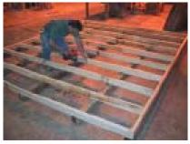
After you have squared the floor, fasten the rest of the 2x4's to the 4x4's.
