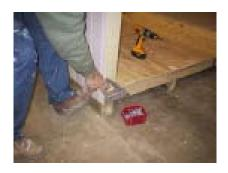
Install section A, keep even with the edge of the floor and push it in against the floor from the outside.
