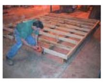
Then place the 4x4 pressure treated runners underneath this frame. Fasten only on the ends.
