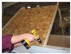
Install first sheet of OSB (orient strand board) sheeting. Fasten only on the bottom first. Refer to layout diagram for your specific building. Use black-headed screws to fasten.
