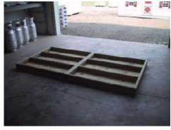
To begin construction of your Cape Cod playhouse simply lay out (2) 4x4 flooring sections side by side. Make sure it is on a level area.
