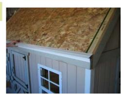
Install drip edge all around the edge of building as shown.
