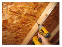
Once the frame is fastened on the outside you can break screws poking through the roof. You can also fasten the frame from the inside out.
