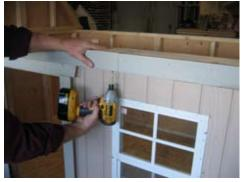
Fasten the 1x3 to the center section using black screws. This will straighten the 2x6 and make it strong.
