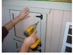
Next install the top door piece. Try to center the door between the header block and the bottom door. If both doors work well, install the rest of the screws and remove spacer bar.
