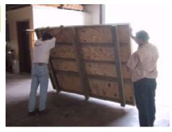
Turn the floor on the back with the plywood facing up. Make certain that the ground is level where the floor sets or you may have problems with the panels or the roof.
