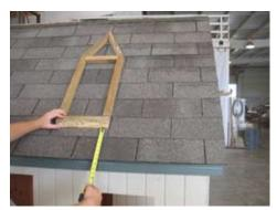
Measure from the bottom up, the edge of the roof to the base of the dormer frame. Make a small pencil or chalk mark once you have positioned the base.
