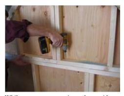
While someone presses in on the outside fasten on the inside. Put 2 1/2" screws on either side of the splices to provide strength.
