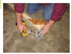
Keep the top of the truss even and install 2 1/2" screws as shown.
