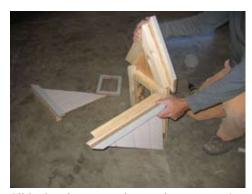
Slide the pieces together as shown. Use  $2 \frac{1}{2}$  screws to fasten together.
