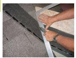
Cut the excess past the dormer. Be sure to use a hook blade so you do not cut into the other roof shingles.
