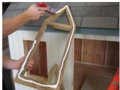
Once you have the correct position apply caulk to the bottom of the base. Make sure it is the bottom!
