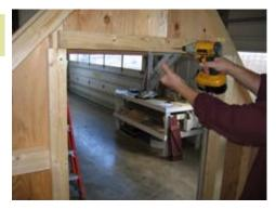
Install (3) 2x3x36" pieces over the top of the door and sides over joints. This will provide strength for the door. Keep even with the edge of the door.
