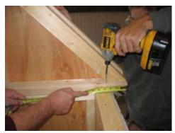
Measure in 5 1/2" from the outside as shown. Be sure to pull in against siding and fasten as shown.
