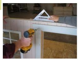
Fasten the other side of the header block B to panel C.
