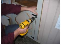
Place the door on the spacer bar. Fasten using only one screw per hinge. This way if adjustments are needed you will not have to undo all the screws. Use black head screw for these.
