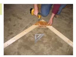
Flip the truss and install gusset on other side.
