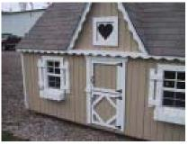
Install the heart window using the small OSB strips. Then install the corner trim using the small white nails. Be careful to not "wrinkle" the corners when installing. Tip: do one side while pressing in, then do the other side.
