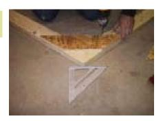
Fasten the truss scabs, keep the top even. Install one scab on either side of the truss. Make sure the scab does not stick out past the truss.
