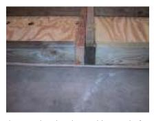
Make sure that the plywood is even before fastening! If it is not you will have an uneven floor, and it could cause problems later.
