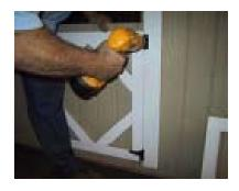
Place door on the spacer bar. Fasten using only one screw per hinge. This way if you need to make adjustments you will not have to undo all the screws.
