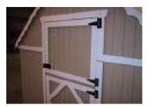
Install the top of the door, centering it between the top door trim and the bottom half of the door. Install the latch.
