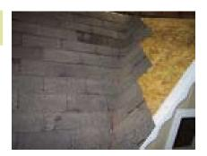
Once you have installed the shingles up the one side, snap a chalk line down the center of the valley.
