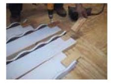
Install (2) 1x3 blocks on the bottom of the 4' 2x6 with gingerbread, the 2' pieces already have the block installed. The 8x10 kit has blocks already installed.
