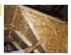
Now have someone hold these in place from the inside. Make sure all 3 pieces of OSB are included with the correct angle of the V-brace to the top of the roof.
