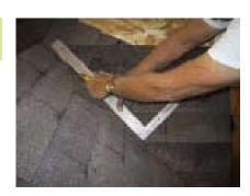
Then install the shingles on the dormer side, then use a hook knife to cut the excess shingles. Do not cut into the next layer of shingles or the roof may leak. Repeat these steps on the other side.
