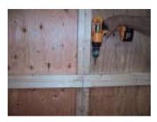
While another person pushes from the outside, fasten on the inside. Be sure to align the top so that it is centered on the bottom wall. Note: the line running from top to bottom. Fasten on all sides of the splice.
