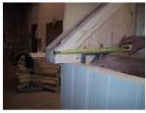
This should measure 5.5 inches from the edge to the inside of the 2x3. The main thing is that it is centered as noted in the previous step.
