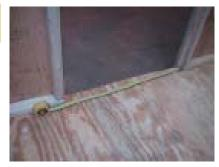
When installing panel L measure the distance between 2x3's. Make sure this measurement is 34". If it is NOT 34", adjust the panels until it is. Otherwise, there will be problems when installing the adult door.
