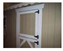
Next install the top dormer piece. Try to center the door between the top trim piece and the bottom door. If both doors work well, install the rest of the screws and remove the spacer bar. 86
