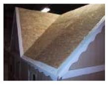
Next install the drip edge (this should have been purchased by the customer at a local home improvement store). You can use tin snips or sidecuts to cut the drip edge and make cuts so that it fits on the angles of the roof. Fasten with 3/4" roofing nails.
