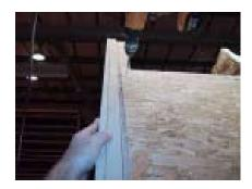
Next install the 4x2 sheet on the front. Note: the same gap between the wall and the sheet as on the back roof.
