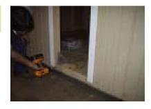
Install small pieces of siding beneath the door. Keep it even with the floor.
