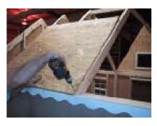
Put a 4x4 (8x12) or a 3x4 (8x10) piece of OSB on the trusses starting with the rear truss. Use black headed screws. It is VERY important to put the roof together correctly, also if your foundation was not level it will show up here!
