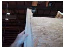
This shows what the edge of this sheet will look like on the end wall. Note: the gap between the wall and the sheet.
