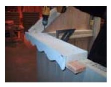
Install the shorter 2x6 with gingerbread, match sets of 4 (8x12) or 3 (8x10) with the numbers and X and O on the pieces.
