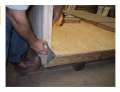
Make sure it is even with the edge of the floor. Push the wall in as shown so that the siding is against the 2x4's on the floor. Fasten the panel onto the floor.
