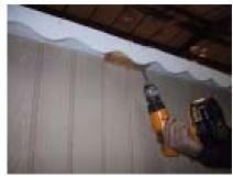
Once the last piece is in place, fasten the blocks underneath to the other piece. This will make the wall and 2x6s sturdy. Repeat the steps on the other side.
