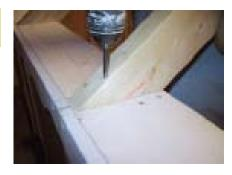
Note: where to place the edge of trusses. Place on the edge of 2x6 and not on the gingerbread.
