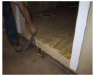
Install the siding beneath the door and put the spacer on top. You may have to screw it in place to keep it from sliding since it is a larger door.
