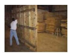
Turn the floor around so that the plywood faces up. Make certain that the ground is level where the floor sets or you will have problems with the panels or the roof. You will need 3-5 people to do this, do this with caustion. Do not allow anyone under the section as is shown in the picture.
