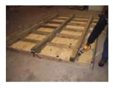
This picture shows the optional 4x4 runners, you will need 3 in order to have one under the center joint. If you use two the floor will sag. Note: these are optional, but will aid in moving the building later. ie: you can put a chain over them and use them to slide over the ground or onto a trailer to move to a different location. If you are adding a deck and rail these are not optional. These allow the small door clearance to open and close.
