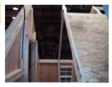
Center the sheet on the other truss that the sheet reaches too. Now fasten this entire sheet, screw roughly 8" apart.
