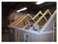
Install trusses in premarked spots. You may have to pull them to the corret position. This is from not fastening the scabs correctly, or from bowing wall or other factors.
