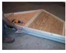
Fasten panels I and J to each other. Make sure they are even on the bottom. Piece may bow slightly; this can be made striaght in the following steps.
