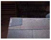
Cut pieces for the ridge cap. See instructions on the shingle package. A regular utility knife works well for this, cut the shingles from the back side. To start with, cut one into a smaller piece as shown. Then install on the top using 7/8" roofing nails.
