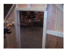
Install (3) 2x3x36 pieces over the top of the door and sides over the joints. This will provide strength for the door. Keep even with the edge of the door.
