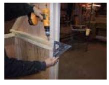
Keep the edge of the door frame even and push the trim in against the siding and fasten. 32
