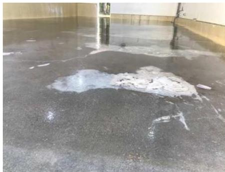
Clear epoxy used as primer / mvb over patch work. Both jobs ready for flake to hide all imperfections in floor.
