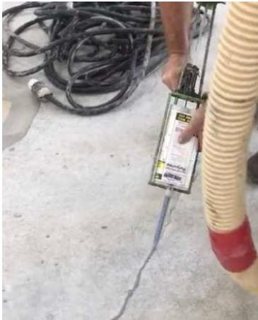
Joints can be pre-filled, then excess grinded off with machine along with rest of floor.
