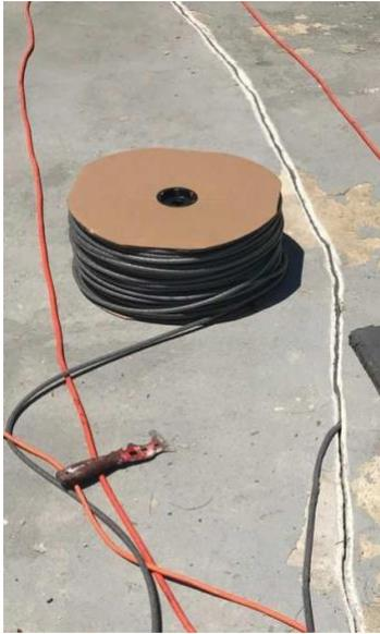
1/4" back rod shown Installed in crack, then filled with polyurea super flexible joint filler.
