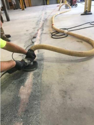
Grinding bondo and pre-flake patch over exceptional wide expansion joints, 1/4" back rod was pre-installed in joint, followed up by polyurea joint filler.
