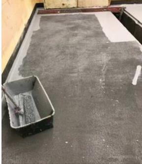
Shown epoxy is rolled 4" up wall always use 6" & 18" rollers.
