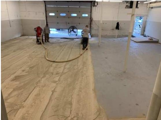
**14-16 grit easily removing failed epoxy for big box store brands**
