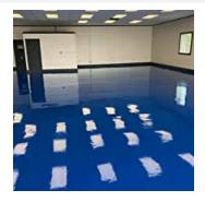
Step 2: Proper Mixing & First coat Application Day 2
