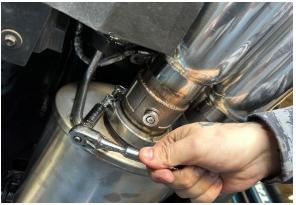
**20.** Mate the v-band flange on the driver valve tip assembly to the flange on the muffler. Align and position the v-band flange so both flanges are fitted within the grooves of the clamp. Reinstall the lock nut and snug the clamp using an 11mm deep socket and 3/8" drive ratchet. The clamp should be positioned with the lock nut towards the inside of the vehicle, the bolt on top and horizontal.
