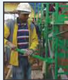
The Jack Handle moves from tower to tower and jacks up the masons and their workbench together.
