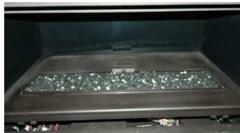
1) Start installing Crystals on the Burner (NG,LP,ULPG)
