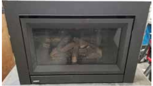
Completed Faceplate & Safety Screen Installation
