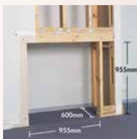
Timber framework partially clad with 12mm Villa Board
