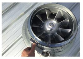
14. If you have a V30 series fan, unbolt the fan flange and use reverts or Tek screw to fix the flange to the ducting
