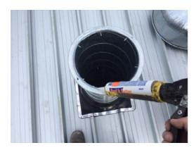
13. Screw and seal rubber boot to tin roof, if tiled roof mould the led to the shape of roof and seal the flashing to the roof tiles.
