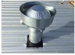
16. Re bolt V30 fan and silicon top of nuts as well as rubber boot making sure it is all water and air tight.
