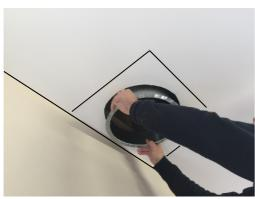
4. Make sure hole cut is big enough and has clearance for the pop to go into ceiling cavity
