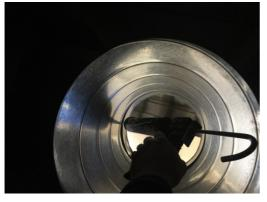
11. Place ducting through the roof and onto the starting pop and silicon the pop to the ducting for air tight seal.
