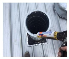
15. Make sure the top of the flange is flush with the top of the ducting and seal the top with normal roof and gutter silicon
