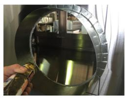
9. Rivet starting pop on to stainless steel flue and silicon with normal roof and gutter silicon
