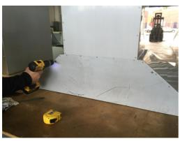
10. Work out wall studs or canter of brick and correspond the measurements to rear of rangehood. Use 12# 50mm long wood screws for timber stud fixing or 10mm diameter 50mm long dyno bolts for masonry/brick wall.
