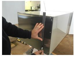
6. Transfer the measurements from the ceiling to the stainless steel flue
