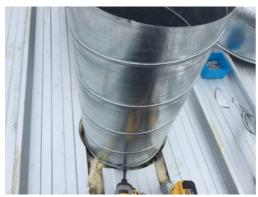
12. Have only 250mm to 300mm of ducting to penetrate through the roof to allow for rubber boot. If you have tin roof, cut some tags and screw to roof and flue for extra support. For tiled roof, wood screw into tile batter or rafter for extra flue support.
