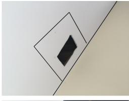
Mark out the flue size on the ceiling and do a small cut out in the plaster to see if there is any obstructions in the ceiling cavity.
