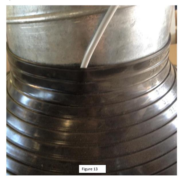
**Step 14:** once cable has been placed inside dektite finish screwing dekite down and silicon all edges
