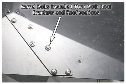
6. Place the larger half of the Barrel Bolt (the one with the large cup washer in Fig.3b) on the outside or top side of the roof, thru the hole, then install the other half (or screw also Fig.3b) into it. Snug but don't tighten down until all 26 bolts are installed into both sections. Fig.3a also shows the bolts installed looking from the "Top side" of the roof as finished.
