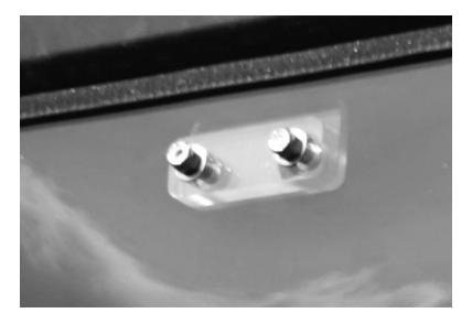
10. On the sides you will use the metal brackets. Take a 1" bolt, washer and run them through the bracket and then through the slot along the sides from the inside out. Then screw on a thumbnut on the outside and tighten down. See the following photos.
