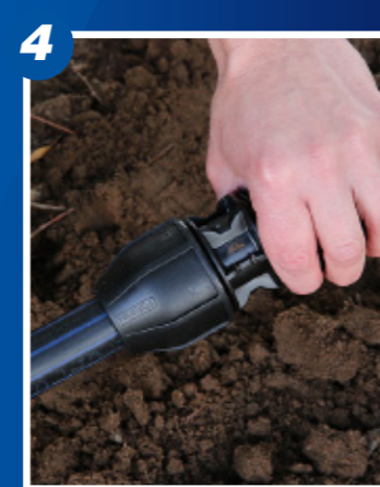
4 Fitting is fully tightened when the nut butts against the flange of the body.
