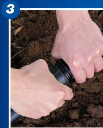
3 Tighten the nut by hand (up to 25mm) or with a wrench.
