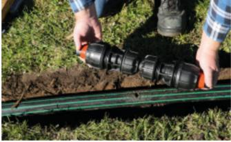
Philmac has released a range of pipe repair kits in common metric and rural sizes.
