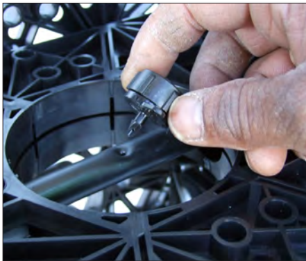
Insert nozzle tightly
