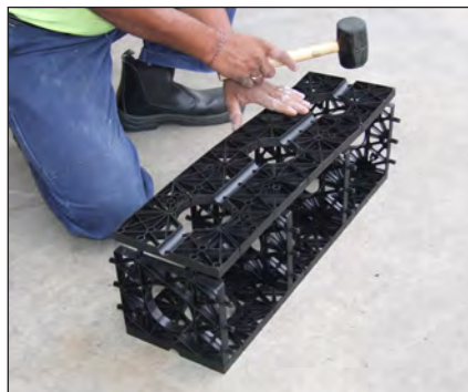
Attach top plate. Ensure the irrigation channel on the long plate faces up.
