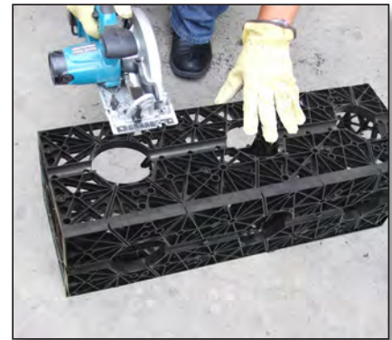
Cutting the module with a circular saw
