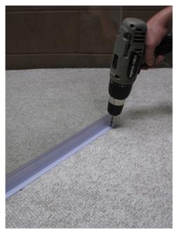
6. Drill a pilot hole and use a screw that is appropriate for the surface you are attaching to. Use four screws per side.
