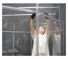
13. Adjust both Lid support bars to the width of the font panels. Rest one support bar on top with the J-hooks at least 4-inches from the edge of the end panels. Place the other bar about a foot in front of the first bar. Do not extend the bar beyond the red limit mark.
