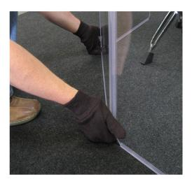
9. Use your fingers to lift the panels at the bottom cable cut-outs to pull or push system into final position. End panels should be parallel and symmetrical on either side of the kit, about 7 feet apart for most applications.
