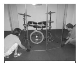
**6.** Use your fingers to lift the panels at bottom cable cut-outs to pull or push system into final position. End panels should be near parallel and symmetrical on either side of kit, 6 to 7 feet apart for most applications. Figure 4 to 5 feet for smaller booths.
