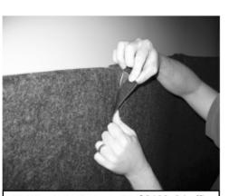
15. If included, move the S2466x2 baffles into position behind kit. Use the Velcro flaps on outside top and bottom sides of S2466x2 to attach the units together. Ends of baffles should overlap inside of shields or butt up against them.
