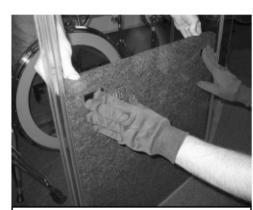
**14.** Place S2224/S2216 baffles in position on shields. Have assistant apply opposing pressure from opposite side then press baffle corners to secure Velcro to shield.
