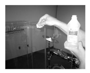
Lubricate the top of the panels with rubbing or other quick-drying alcohol solution to aid installation.
